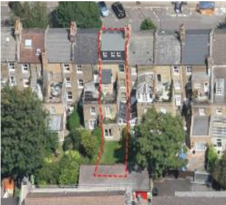
Image 2 Aerial view from the west
